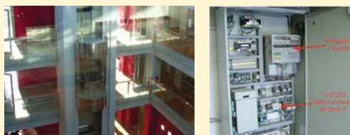
Frequency inverter for 3 phase AC motor (lift-elevator)
