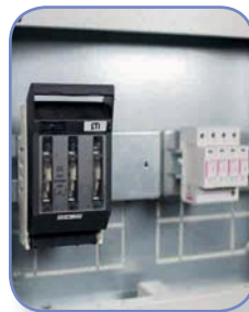
LTL00 disconnector and modular equipment
