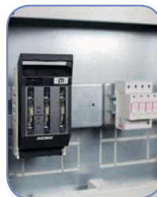
LTL00 disconnector and modular equipment
